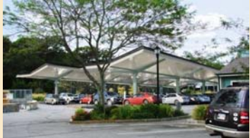
[Figure 4.263] Solar panels over surface parking saves energy and provides shade.
