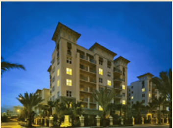
[Figures 4.218, 4.219 & 4.220] Development in the Downtown continues to positively transform the City into a live, work and play environment with street activity that supports transit, biking and walking.
