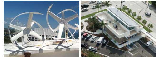
[Figures 4.266 & 4.267] Left: Wind turbines on top of a hotel at Fort Lauderdale beach. Right: a LEED Certified bank near Downtown Fort Lauderdale.
