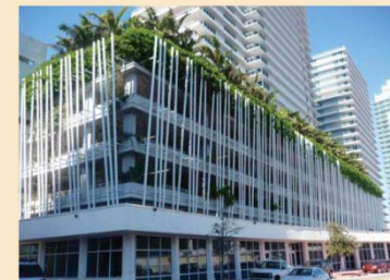
[Figure 4.254] A parking garage with sophisticated styling, screening, windows and green roof elements integrated into the design.
