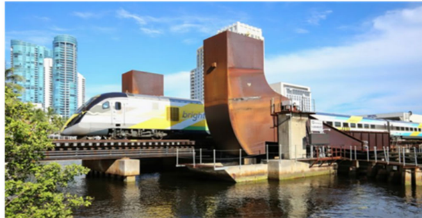
Exhibits 1, 2 and 3 – Photos of Existing Bascule Bridge over New River
