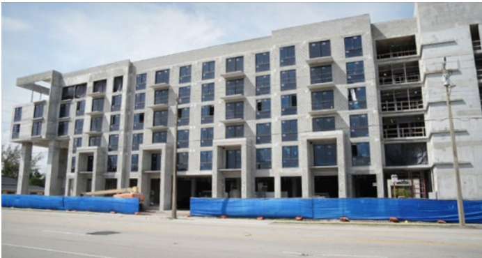
Construction of the The Adderley
