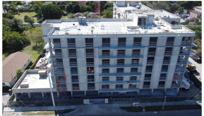
Construction of Mount Hermon Apartments
